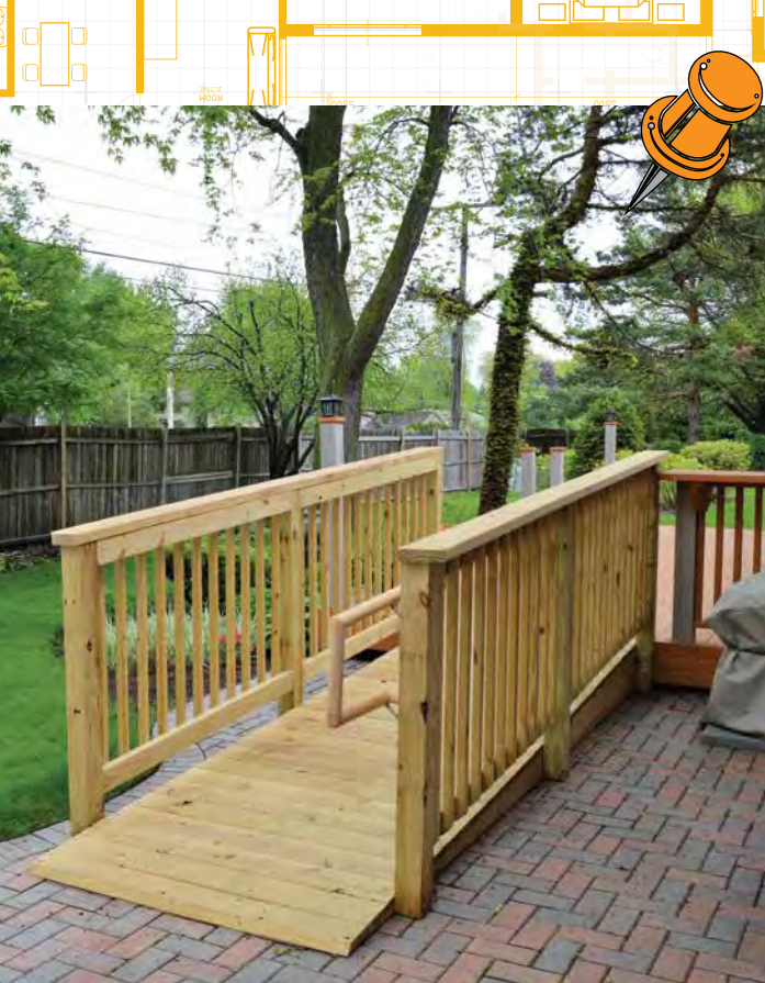
Ramps are a frequent exterior modification. Their slope should be determined by the abilities of the user, however, not by minimum regulations.
