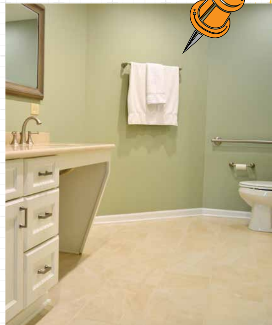
Bathroom modifications may include a cutout below the sink for wheelchair access. The open space allows for wheelchair maneuvering, with strategically placed grab bars.
